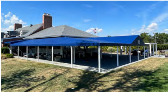
Essex CC Structure with retractable screens
